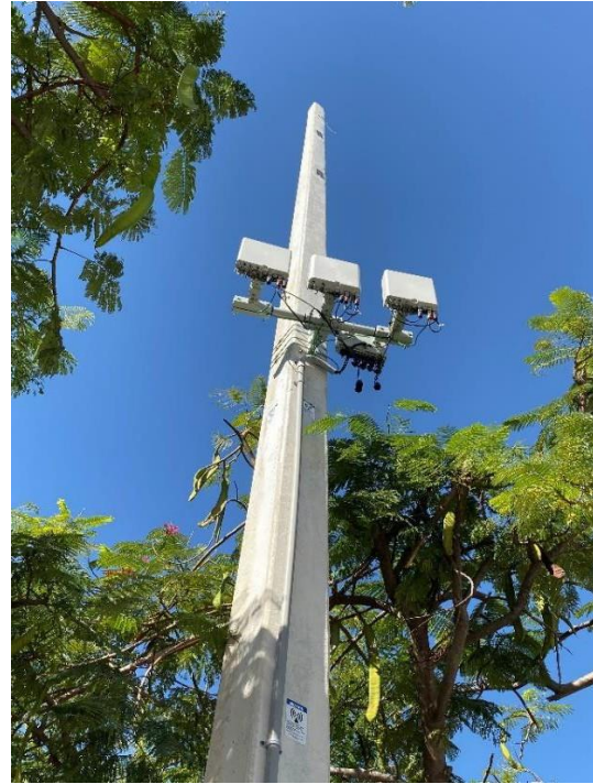
Single-carrier small cell pole
